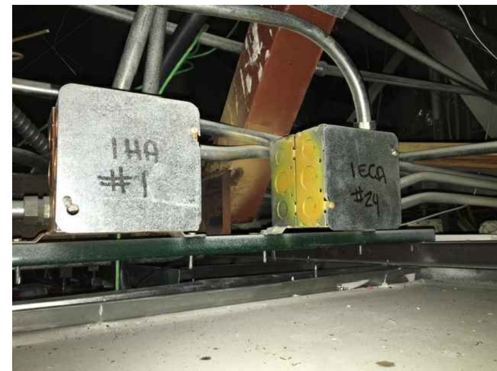
EXISTING J-BOX FOR CIRCUITS 1ECA-24 & 1HA-1 TO BE DISCONNECTED & REMOVED INCLUDING CONDUIT & WIRES TO EXISTING LIGHT FIXTURES
