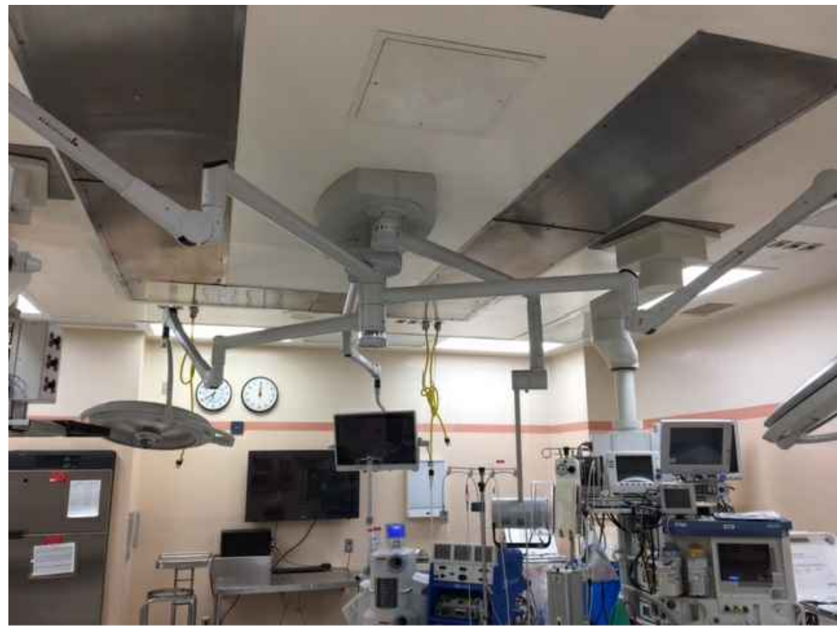
EXISTING SURGICAL LIGHT FIXTURES TO BE DISCONNECTED & REMOVED (EXISTING ACCESS PANEL IS ON LEFT)
