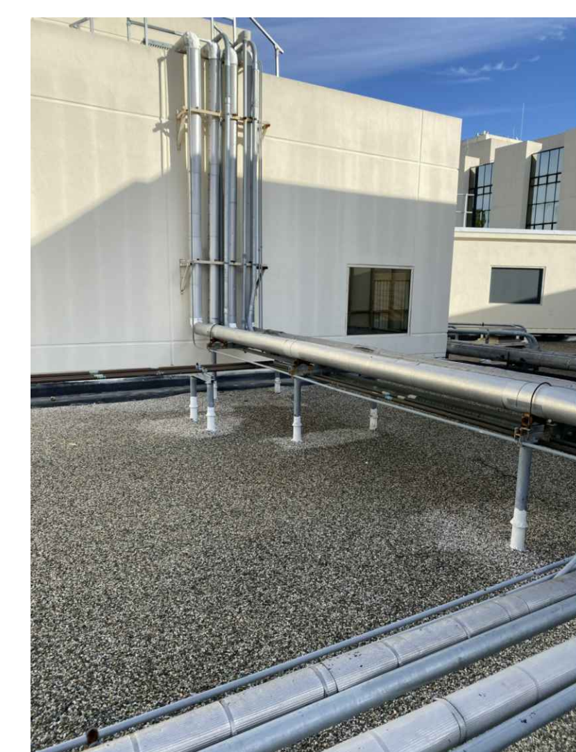
IMAGE 1 - VERTICAL CONDUIT RACK FROM 1ST FLOOR ROOF TO 2ND FLOOR ROOF
