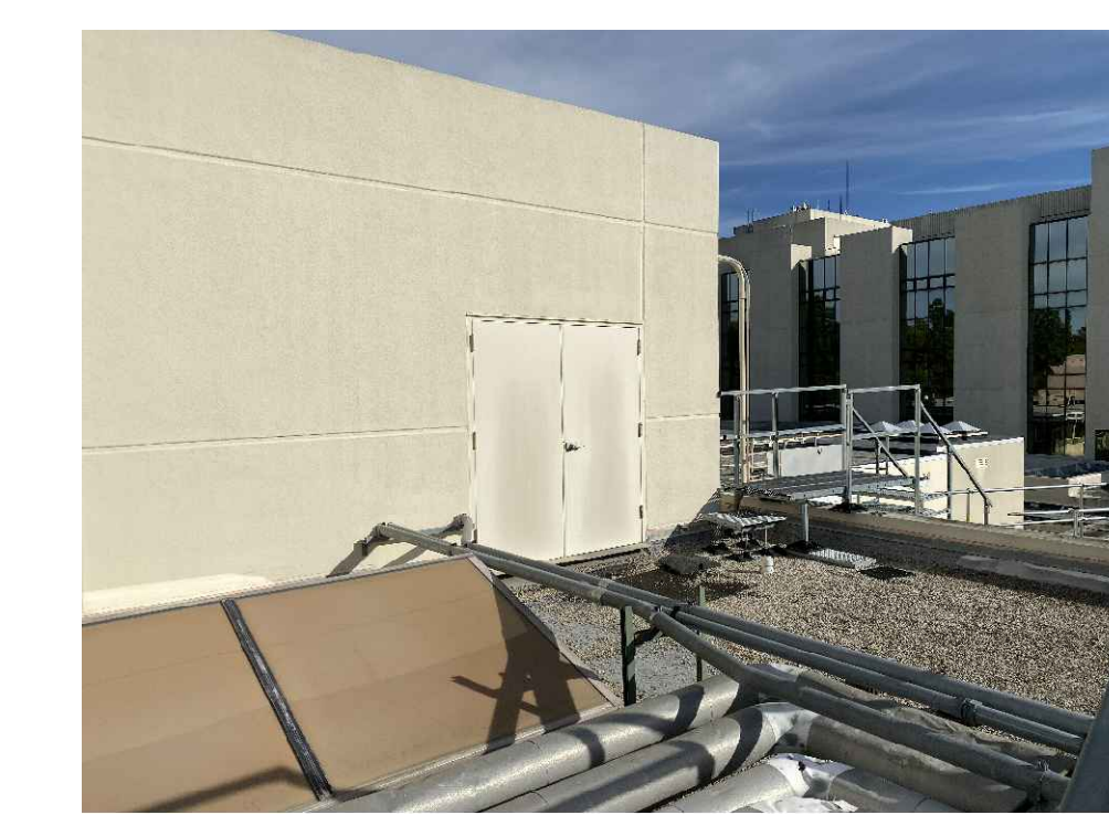
IMAGE 1 - HORIZONTAL CONDUIT RACK @ 2ND FLOOR ROOF
